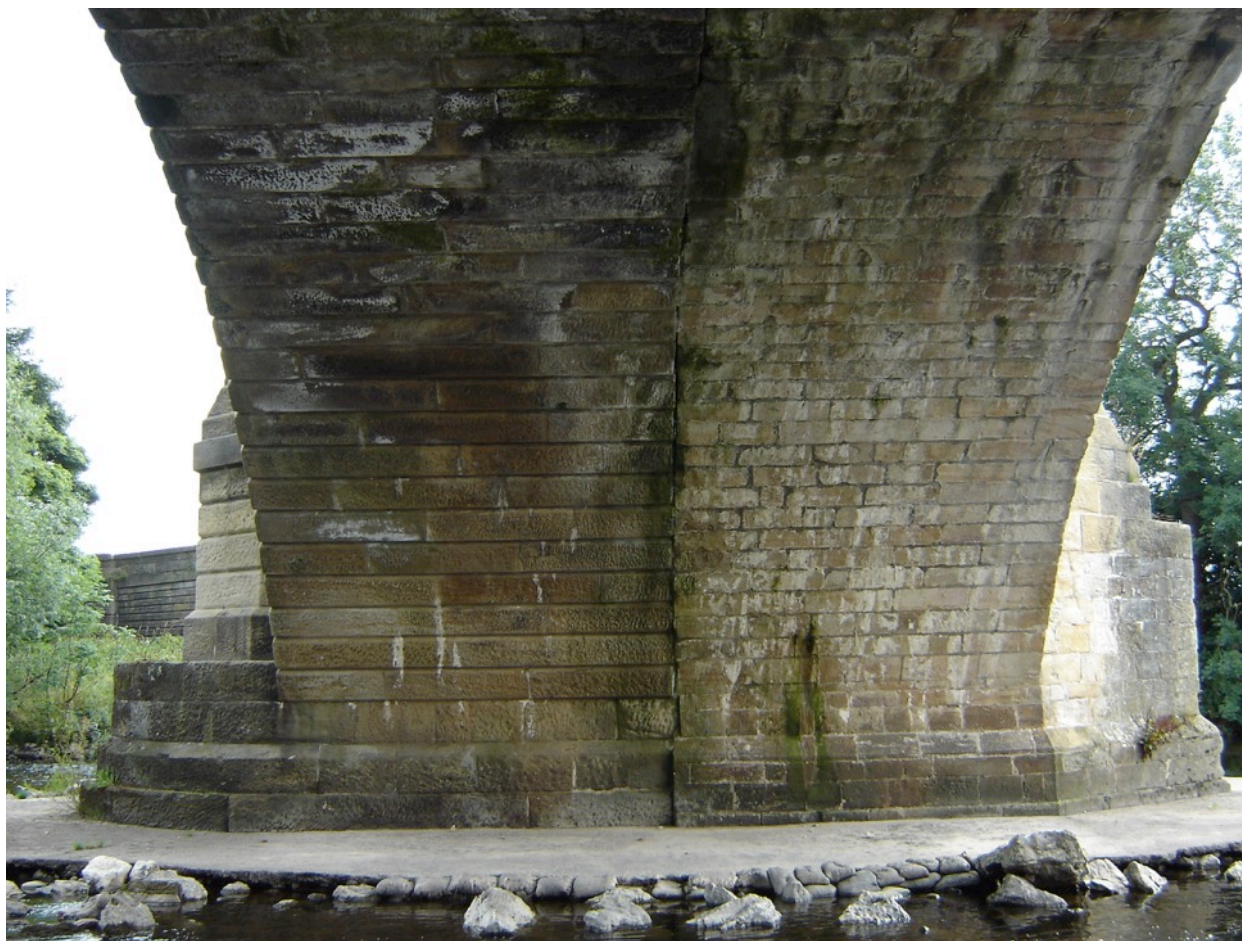
Figure 16 The underside of West Tanfield Bridge showing the older (right hand side) and newer (?1842) parts of the bridge. © J. Buglass.
