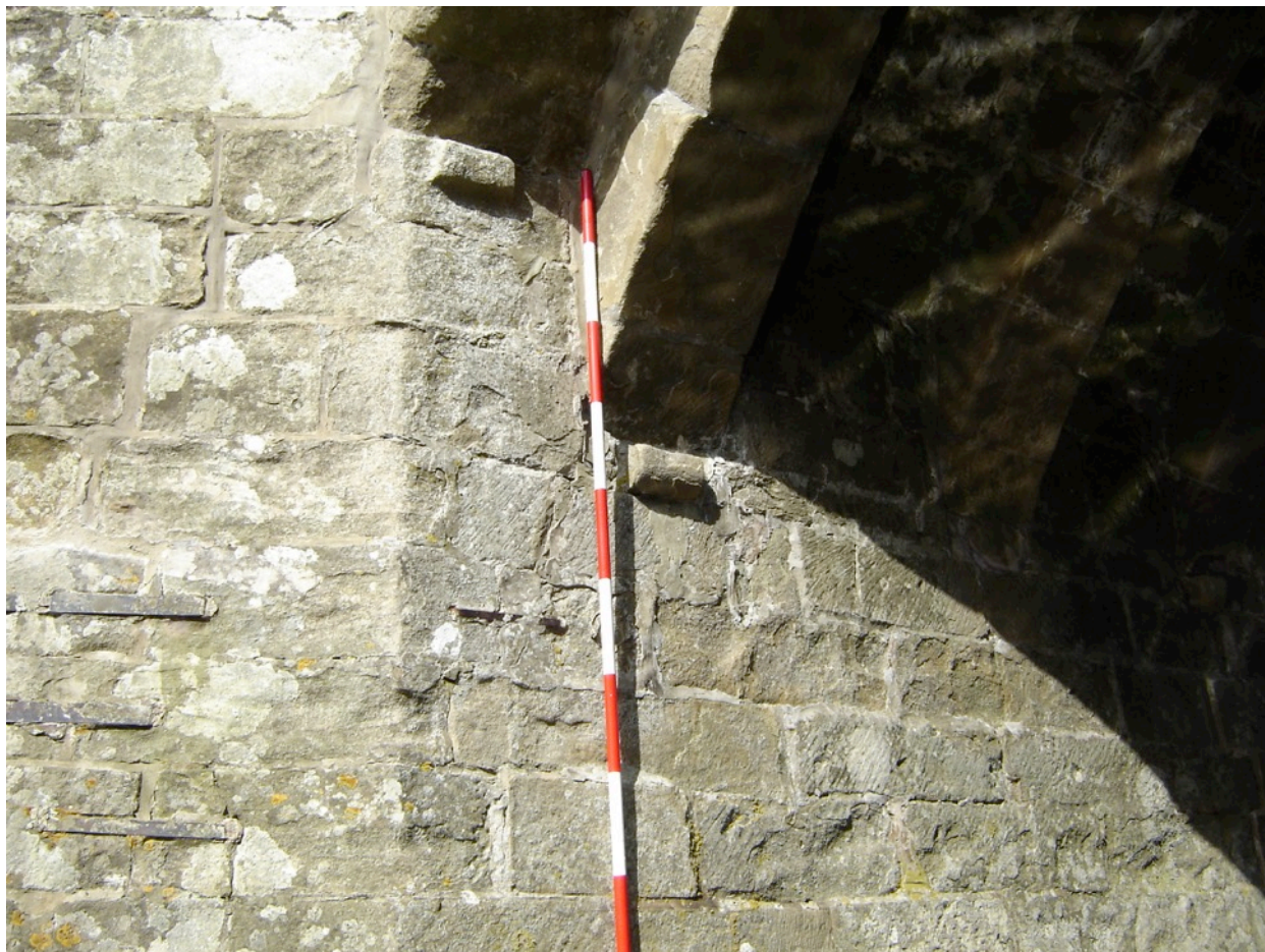
Figure 3 Different height corbels on Arch 3. Scale: 2m. © J. Buglass.
