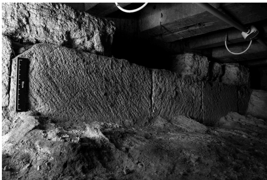
Figure 6 Photograph showing tooling on east part of northern wall. © York Archaeological Trust.
