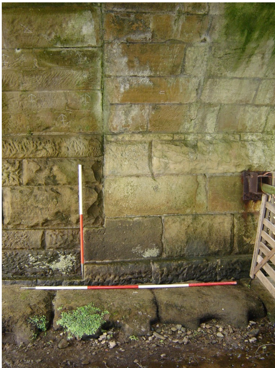
Figure 9 The old (right hand side) and new (1715) parts of Low burn Bridge. Scale: 1 and 2m. © J. Buglass.
