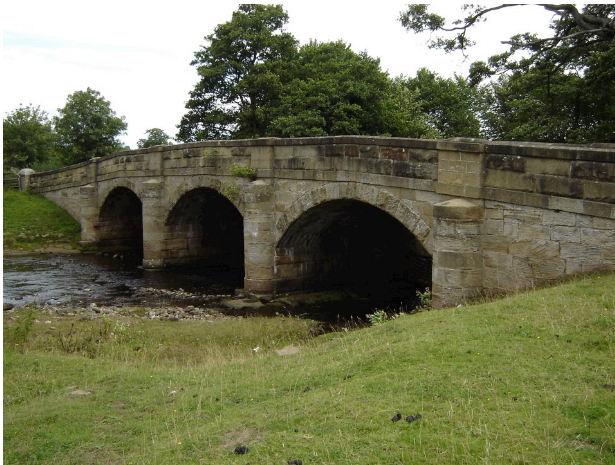
Figure 8 Low Burn Bridge from the west. © J. Buglass.
