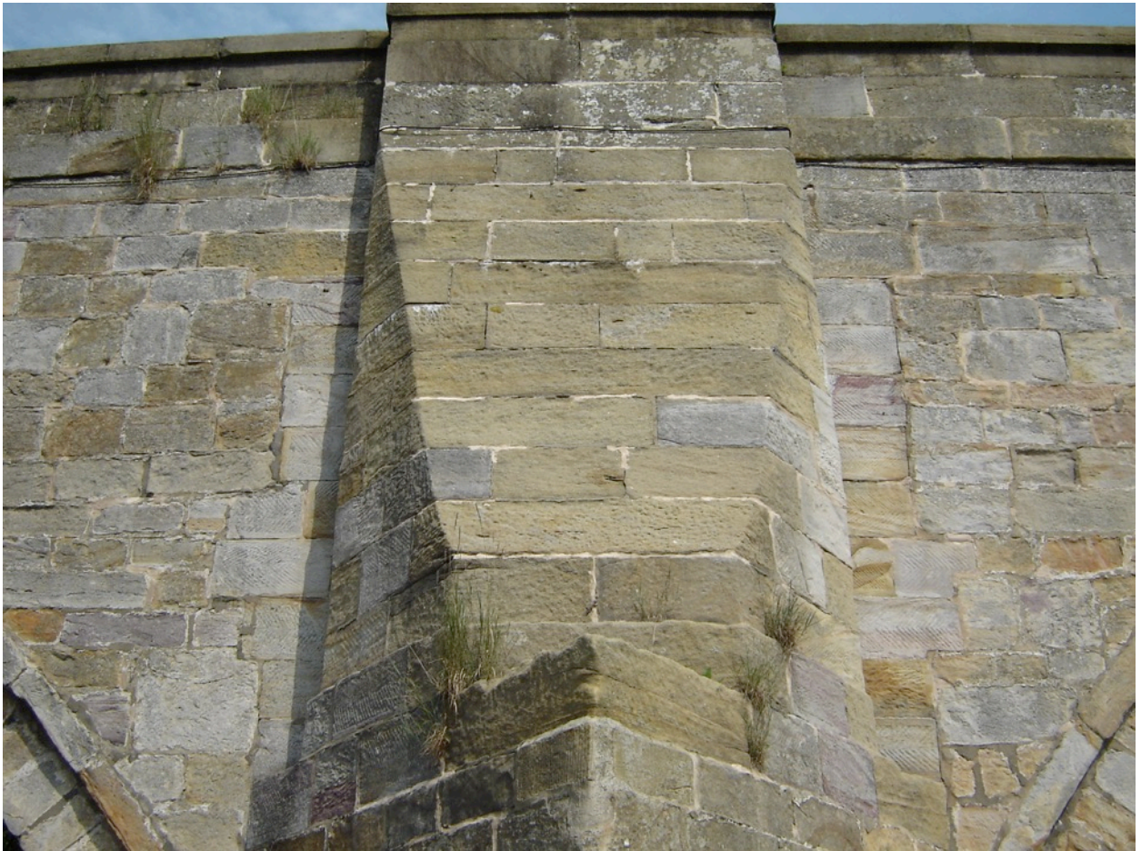
Figure 13 Butt joints either side of the northern most buttress on the western side. © J. Buglass.
