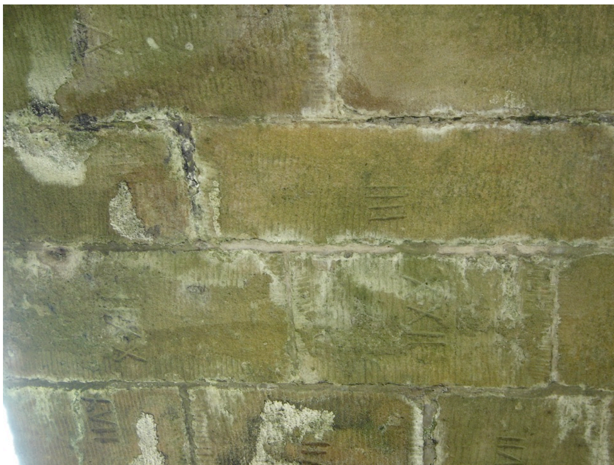
Figure 10 Roman numerals on the underside of the old portion of Low Burn Bridge. © J. Buglass.
