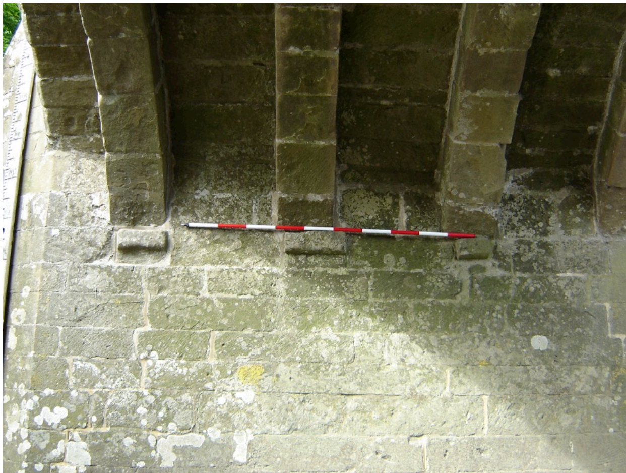
Figure 2 Corbels below springing point on the north side of Arch 2. Scale: 2m. © J. Buglass.
