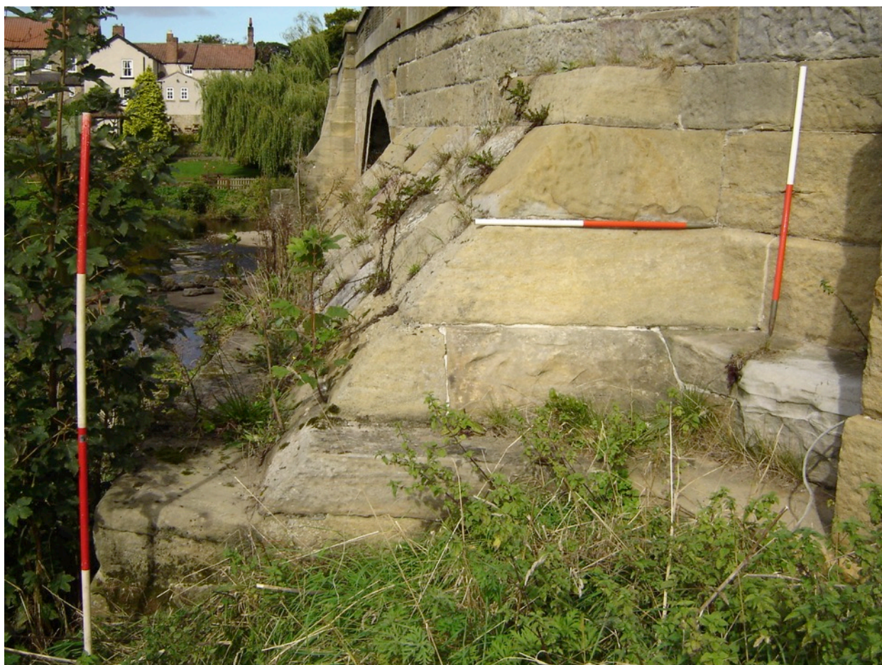
Figure 14 Unusual stone structure on the south-west side of West Tanfield Bridge. Scale: 1 and 2m. © J. Buglass.
