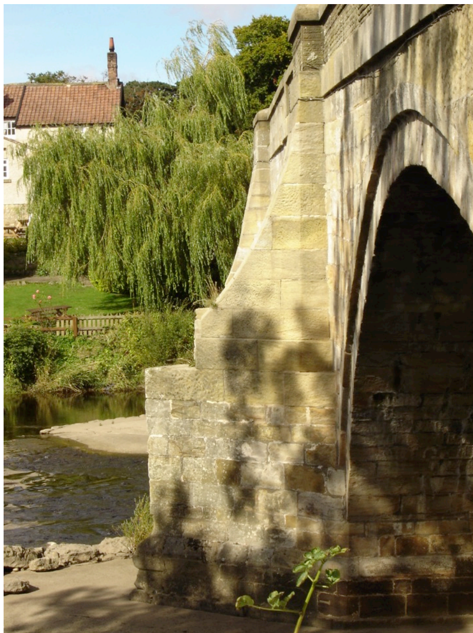
Figure 12 West side of West Tanfield Bridge, looking north showing the differences in the two buttresses. © J. Buglass.
