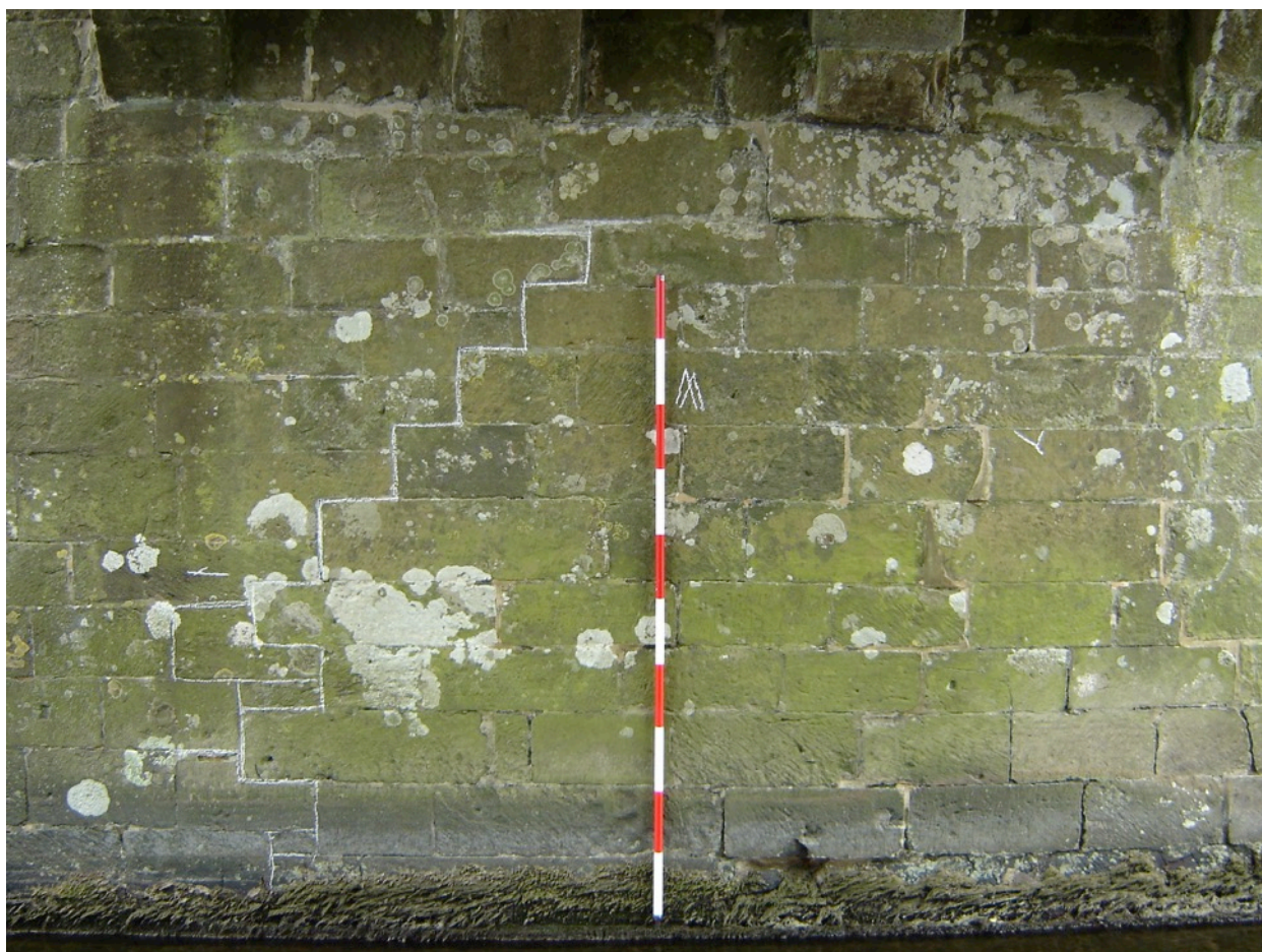
Figure 6 South side of Arch 4 showing the marked change in the stone courses. Scale: 2m. © J. Buglass.
