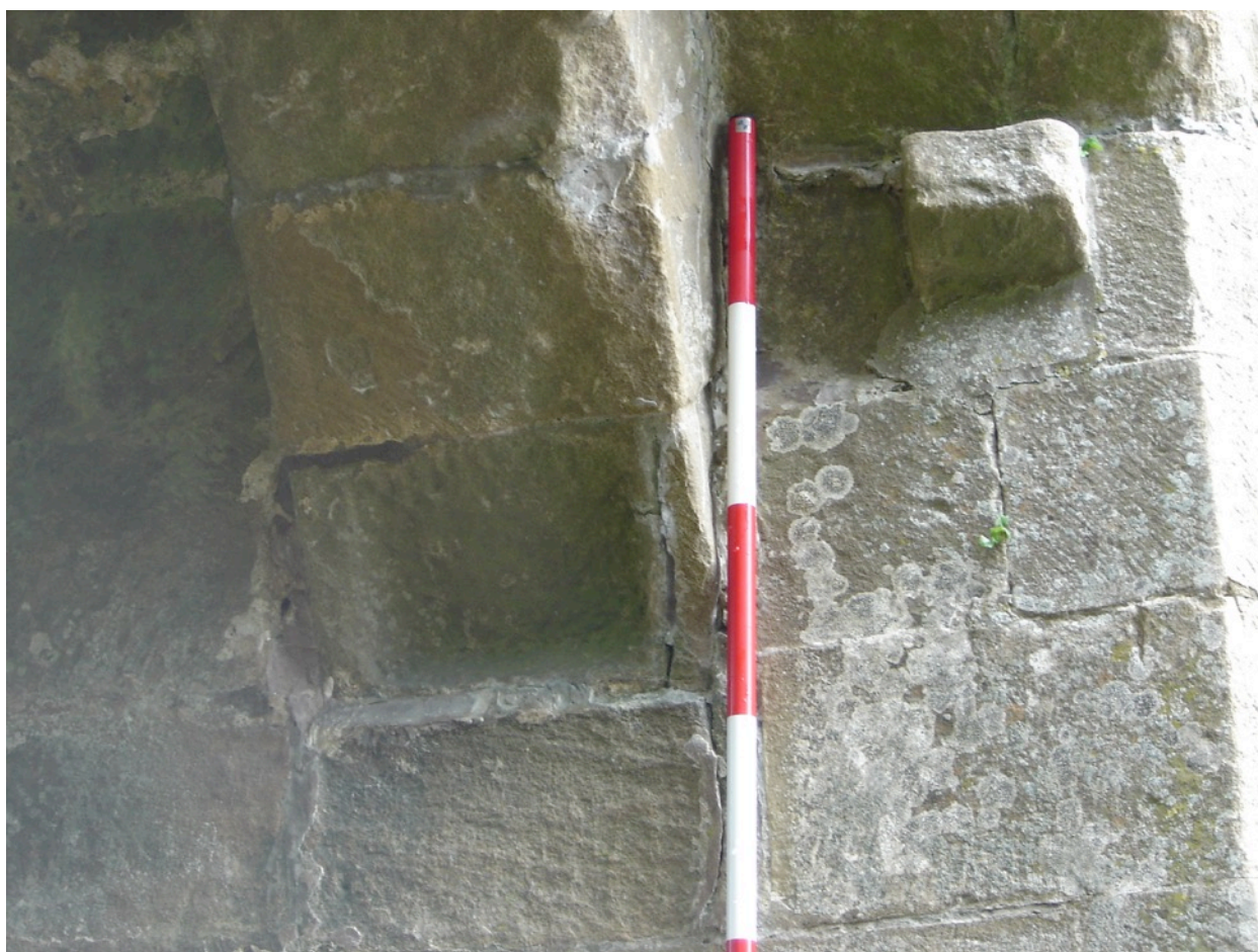
Figure 5 High level corbel and recess cut under the springing point in Arch 3. Scale: 0.1m units. © J. Buglass.
