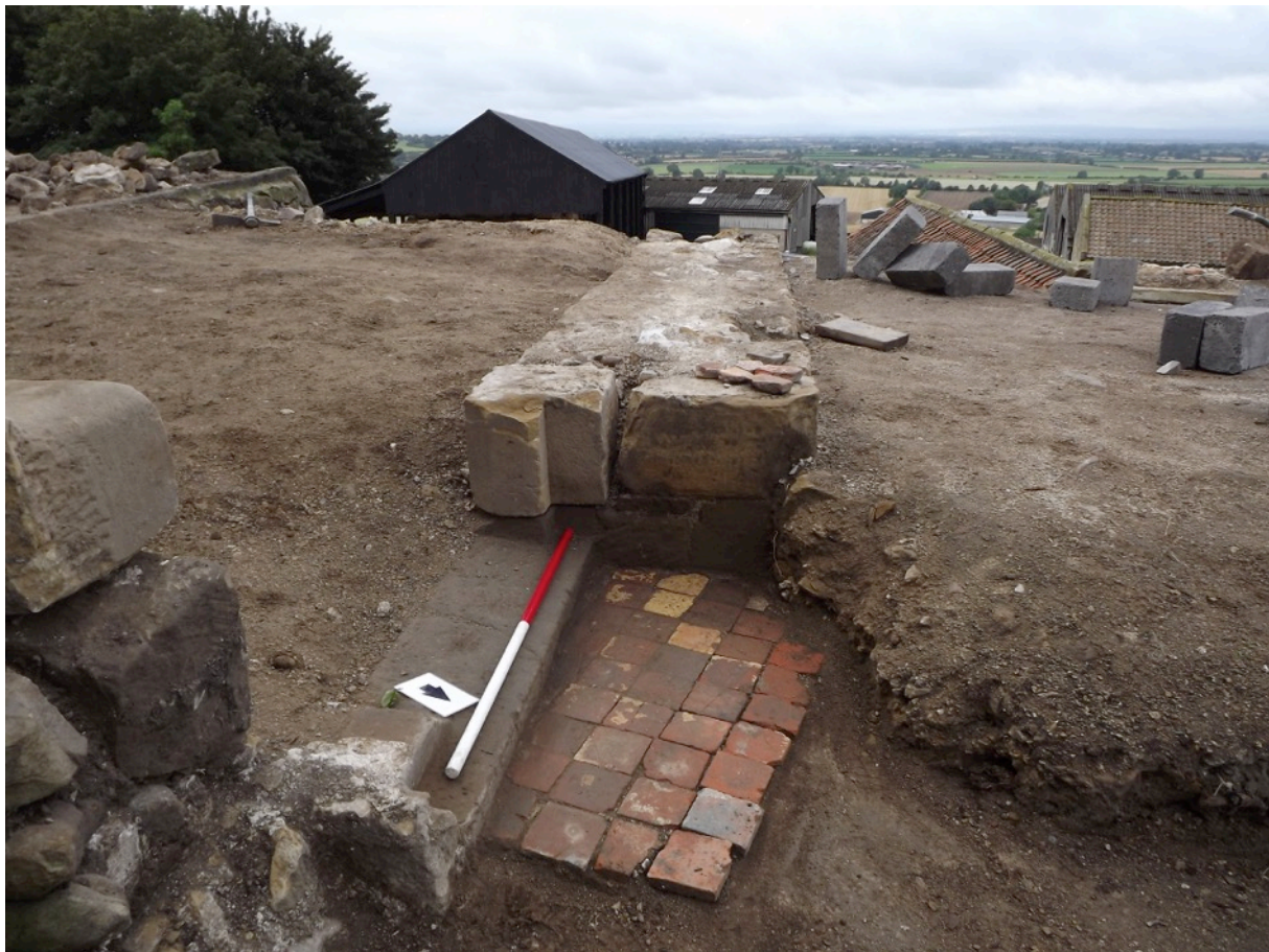
Figure 7 Harlsey Castle, in situ late medieval/early post medieval tiles on upper floor, looking west. Scale 1m. © J. Buglass.
