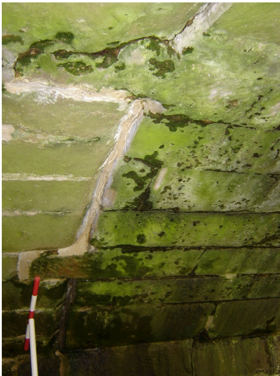
Figure 4 Butt joint in the different phases of the bridge seen under Arch 6. Scale: 0.5m. © J. Buglass.
